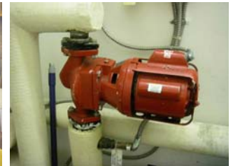
CIRCULATING/RECIRC. PUMPS
