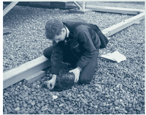
Roof drain cleaning.
