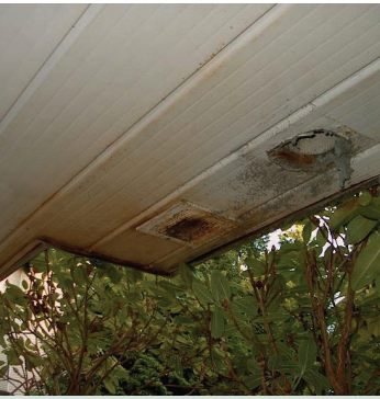
The build-up of debris or dirt on the underside of the balcony limited the air flow through the vent, resulting in damage.
