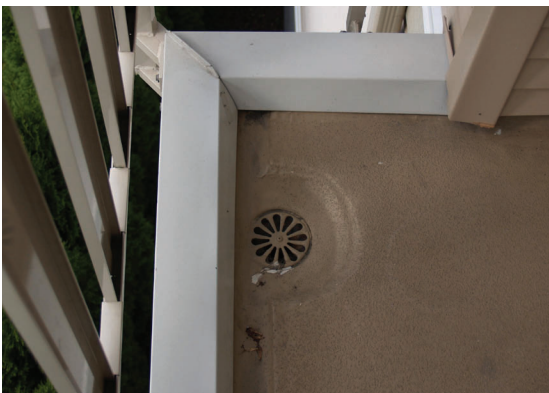
Maintain drains free of obstructions, dirt or debris to ensure they are free flowing and to prevent water ponding.
