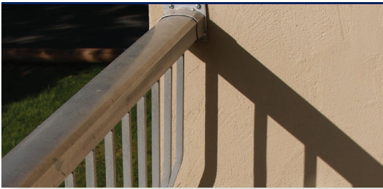
Guardrail connection to the wall can be a vulnerable point of water ingress.
