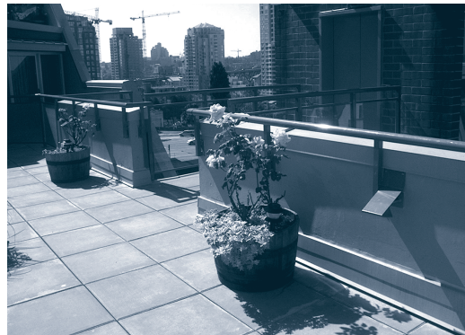
Deck with combination of guardwalls and guardrails.
