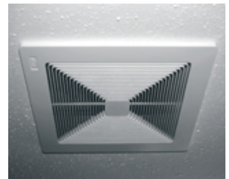
Use bathroom fans, and humidistats if you have them, while bathing or showering.
