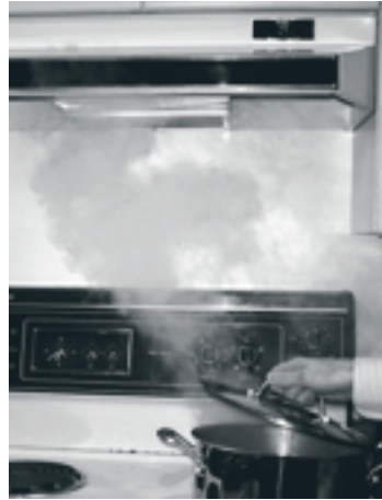
Use your kitchen exhaust fan or range hood to remove humidity generated by cooking. The exhaust fan should be vented to the outside.
