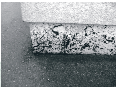
Some coatings such as this acrylic stucco coating over tar-based damp-proofing are incompatible, resulting in a cosmetic detracting instead of providing protection.
