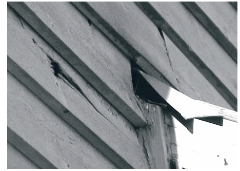
This wood siding has suffered irreparable, permanent damage that cannot be corrected by further paint or stain application. This could have been prevented through proper maintenance.
