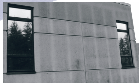
Proper cleaning and renewal of acrylic stucco colour coatings can be required to maintain an acceptable appearance in unprotected areas.
