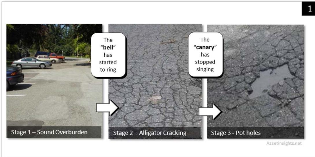
When asphalt paving is first installed it is in good condition. After a few years of exposure and use, minor cracks form. Eventually, potholes and subsidence will occur. The ***bell started to ring*** when the first cracks in the roadway appeared and the ***canary stopped singing*** when the potholes appeared.
